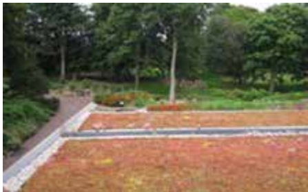
Extensively green roof—Botanic Gardens
