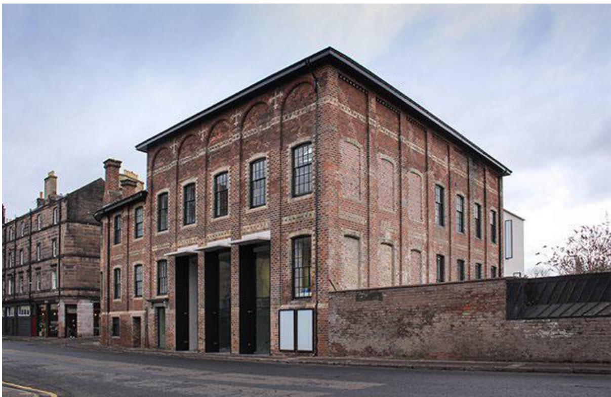
Reusing an existing building— East Market Street Edinburgh Printmakers Gallery
