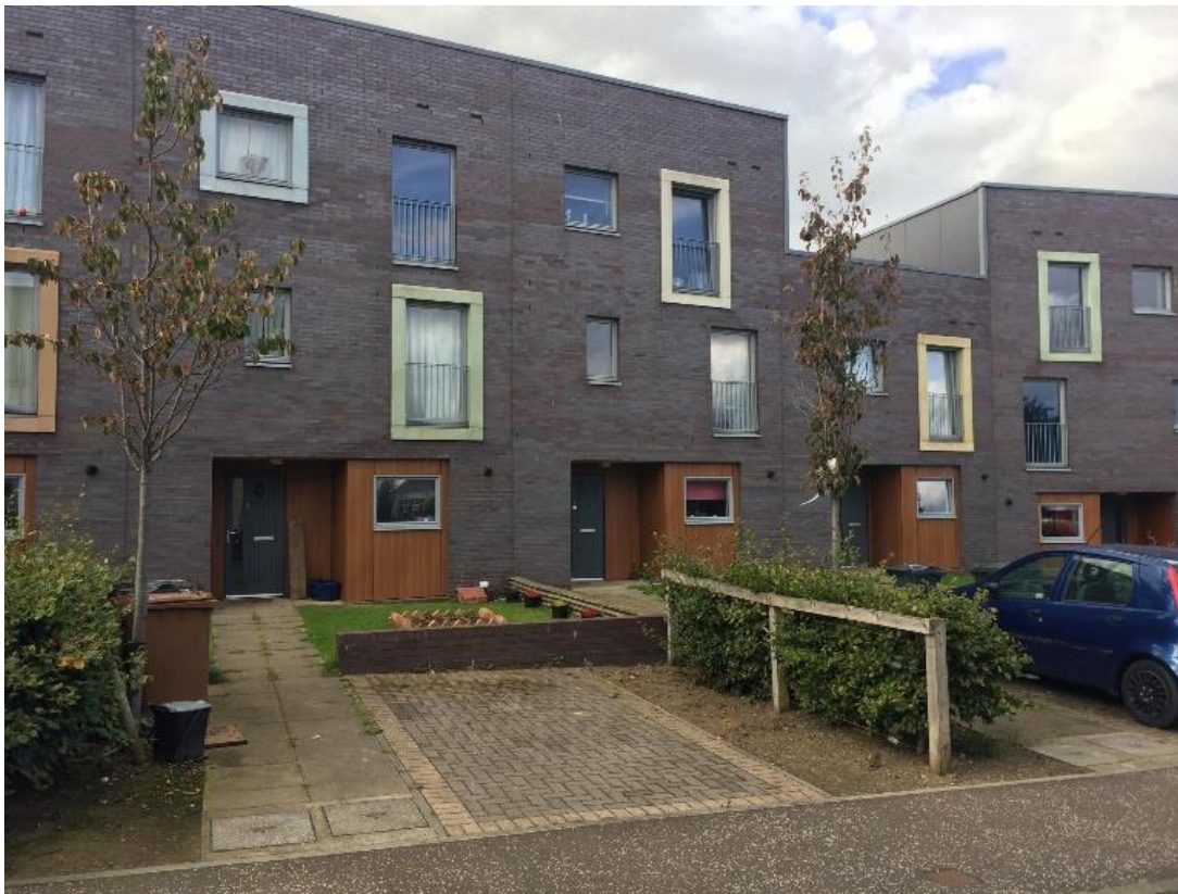
Terraced housing—Wauchope Terrace
