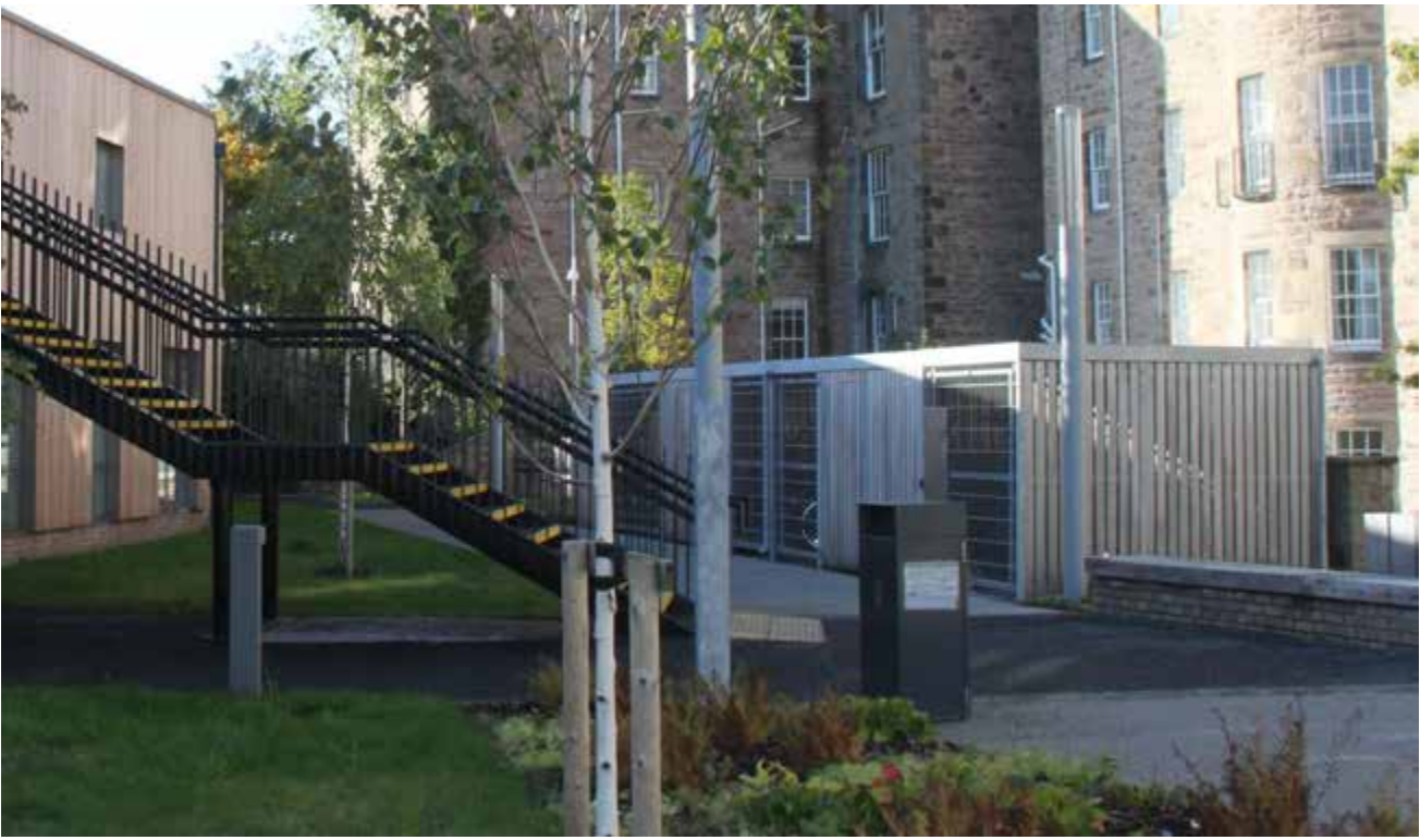
Long stay cycle parking, image c/o Paul Downie, Falco Buccleuch Place Lane Student Housing
